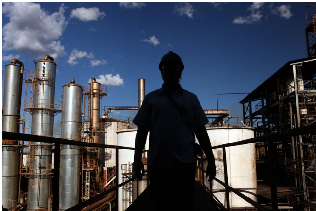
A worker walks next to distilling tanks at the Louis Dreyfus Commodities' Biosev sugarcane processing facility unity near Sertaozinho, Brazil Photographer: Dado Galdieri
